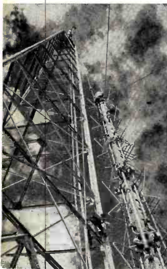
SUPER turnstile for KECA-TV Los Angeles is raised to top of the 303-foot supporting structure. Tower for the ABC video station is on crest of Mt. Wilson, 5,999 above sea level.
